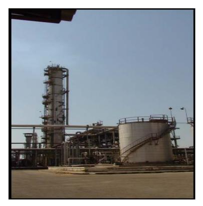
Figure (32): Distillation unit
